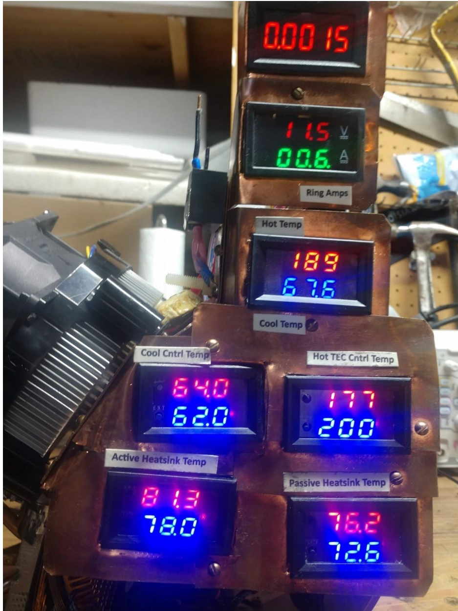
Figure D7. Front of ring after reaching max temperature (two 6-amp heating TECs)
